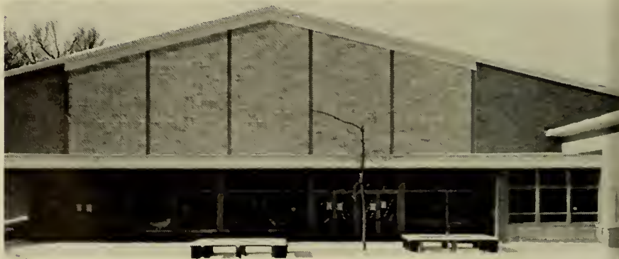
This new $913,000 gymnasium-auditorium-natorium at Drew University was opened Jan. 27. Under construction for one year, it is the largest building on campus and has facilities for physical education, large assemblies, and social events. The main floor seats 1,000 persons for athletic events and has space for 1,200 chairs. The natorium along one side of the main section houses an intercollegiate swimming pool.
